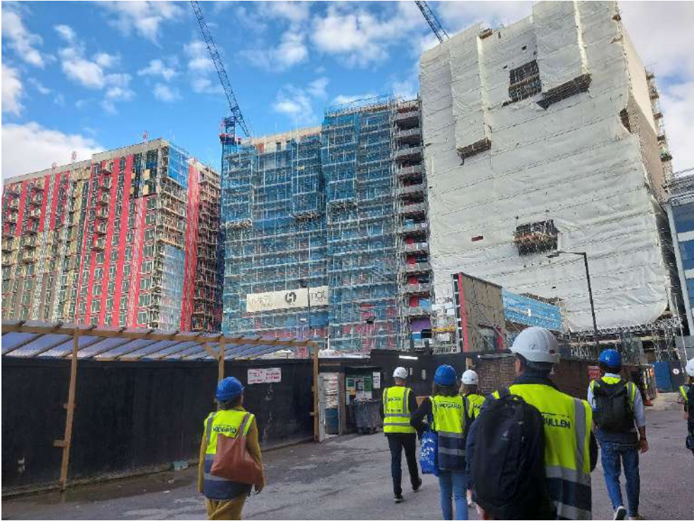
Figure 48. Group visit to construction site
