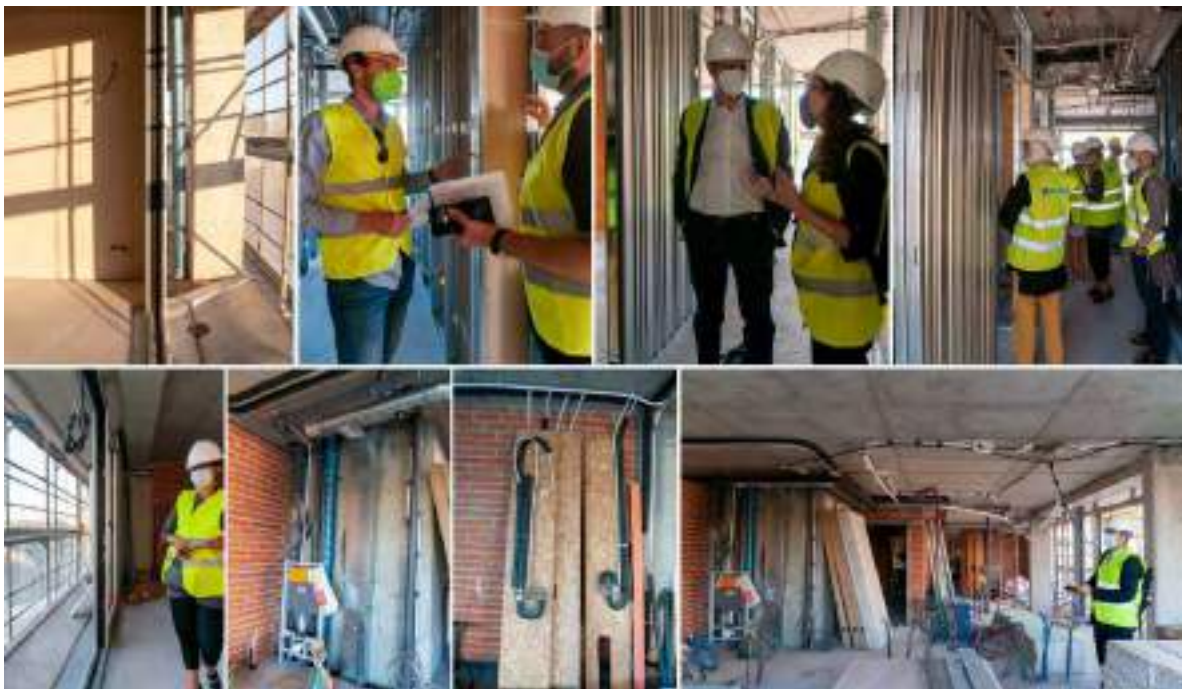
Figure 28. CASAIS session - Visit to a construction site
