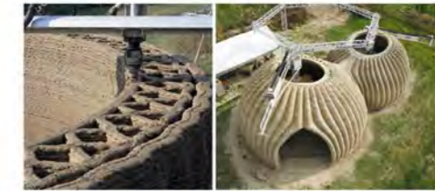
3D House with clay in Italy, 2021 by Tecla and WASP
