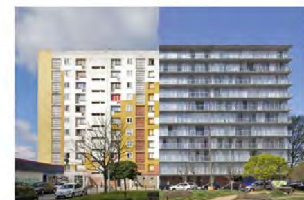
Extensions to preexisting buildings - Lacaton & Vassal, France
